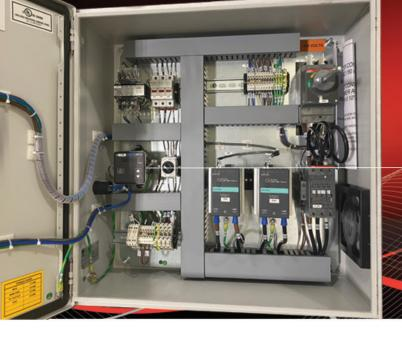
Closed-loop heater control with digital temperature controller
