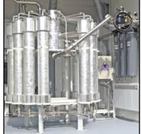
Air Separation & Gas Regeneration CAST-X Heaters fit membrane-based nitrogen production systems, TSA style PPUs, plus several regeneration and dehumidifying processes.
